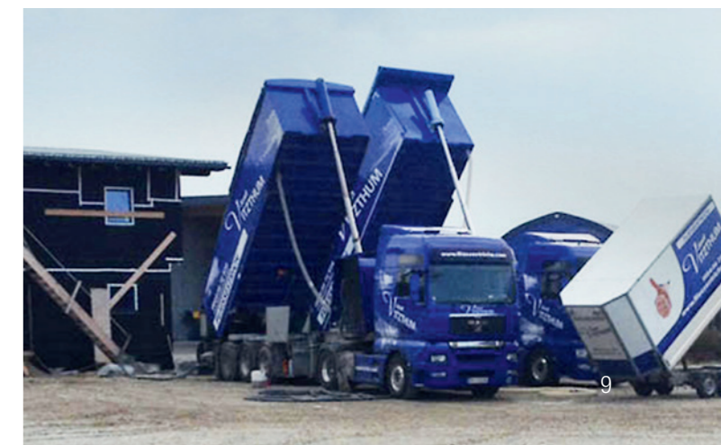
Site with polystyrene pour-in insulation
